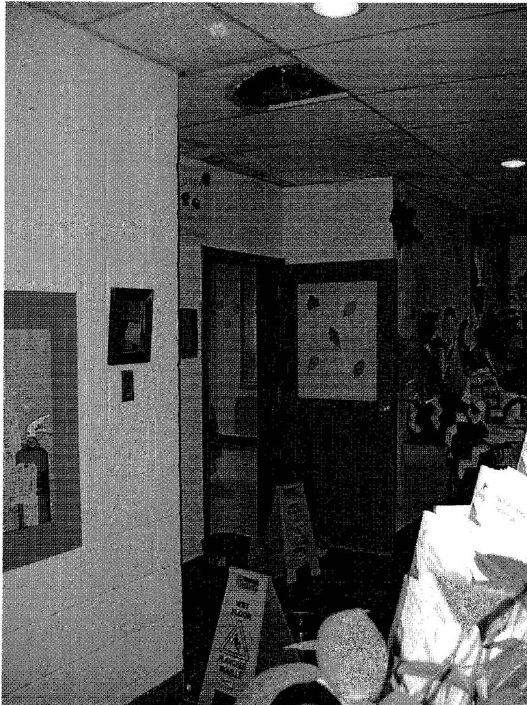
Picture 1: Drop-in Centre reception corridor.
